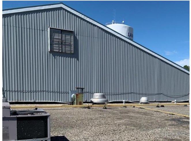
General view of the metal siding on the upper portion of the south elevation.
