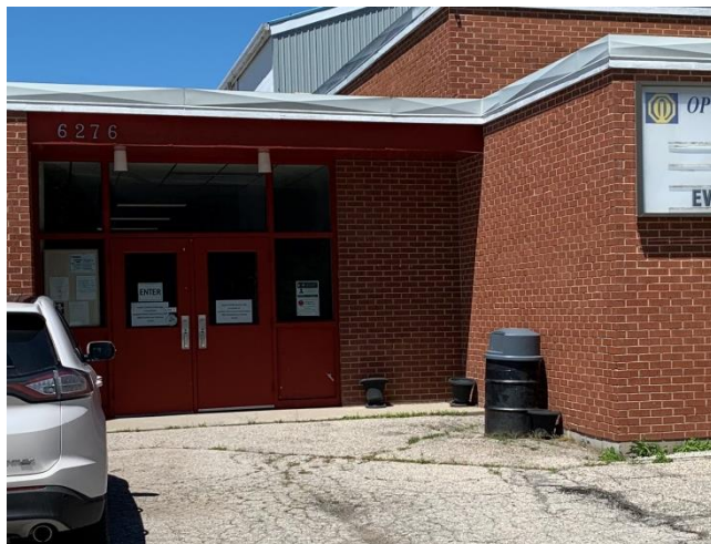
View of the main entrance doors on the south elevation.
