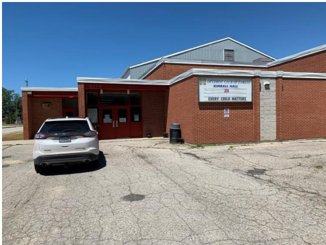
Deteriorated asphalt pavement on the south portion of the site.
