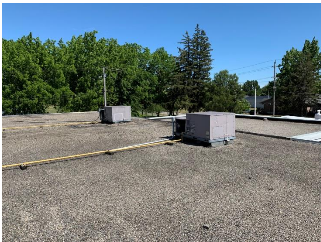
General view of the BUR system on the south roof.
