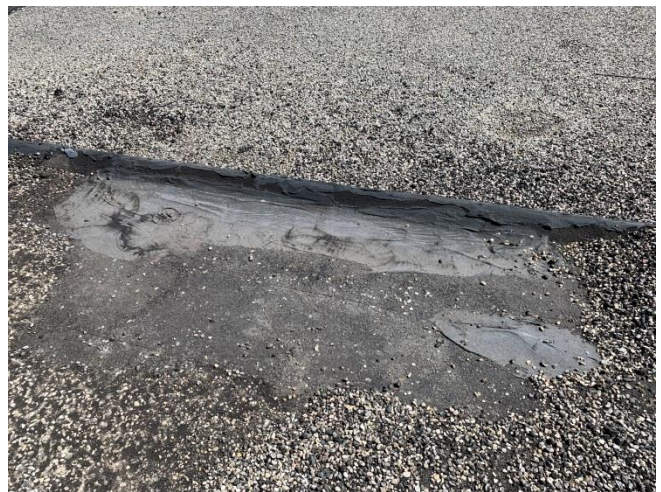
A repair patch on the BUR system.
