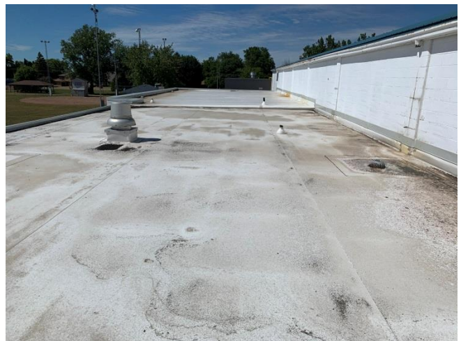
General view of the TPO membrane on the east roof.
