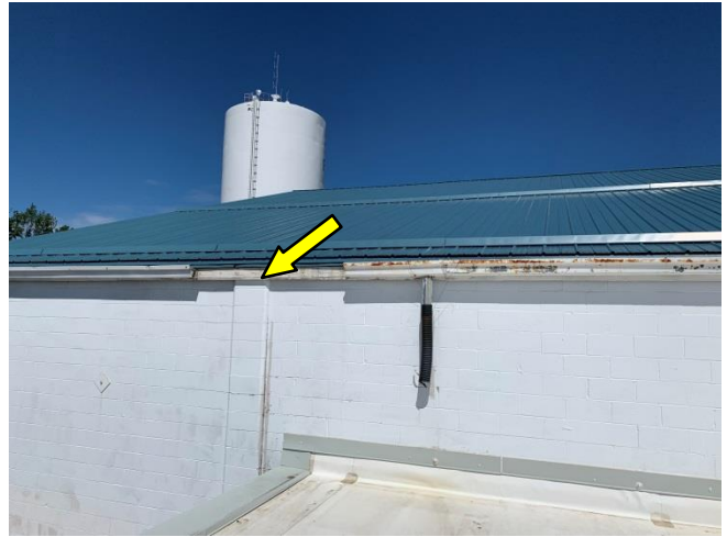
The sloped metal roof was noted to be in fair to good condition.
