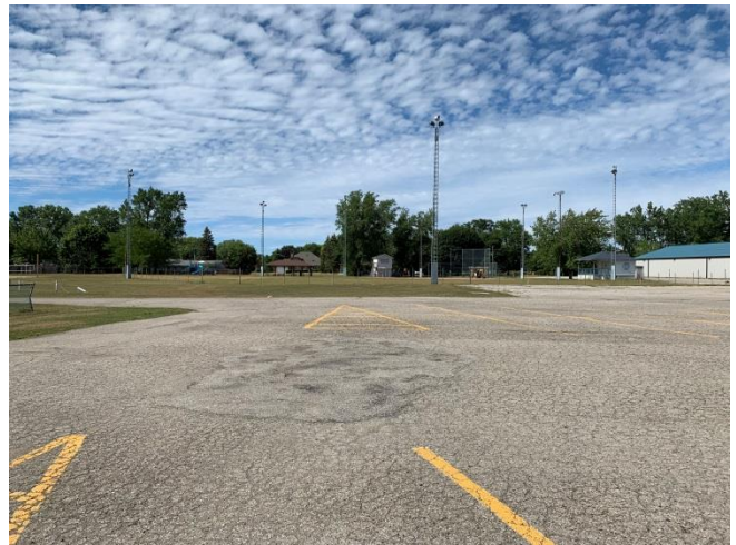
Deteriorated asphalt pavement on the east portion of the site.
