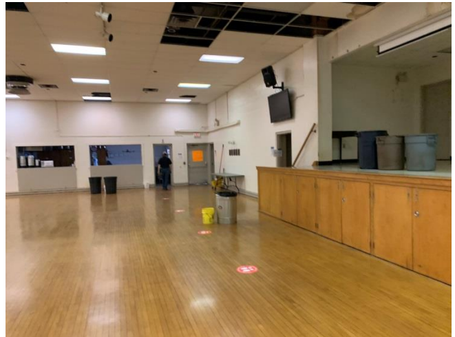
Community hall flooring was noted in fair condition.
