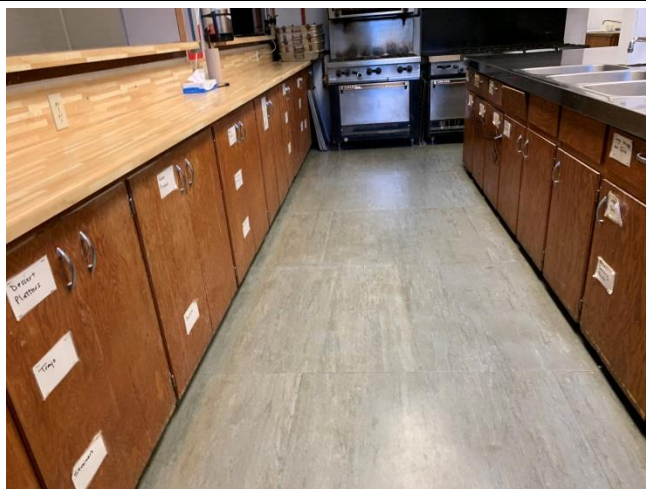
Fixtures within the community hall kitchen appeared to be in good condition.
