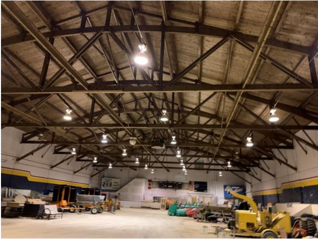
Interior view of the structural elements at the arena.
