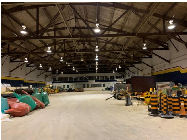
Interior of the arena currently used as a storage area.
