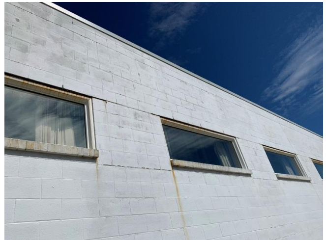
Exterior view of the windows on the west elevation of the building.
