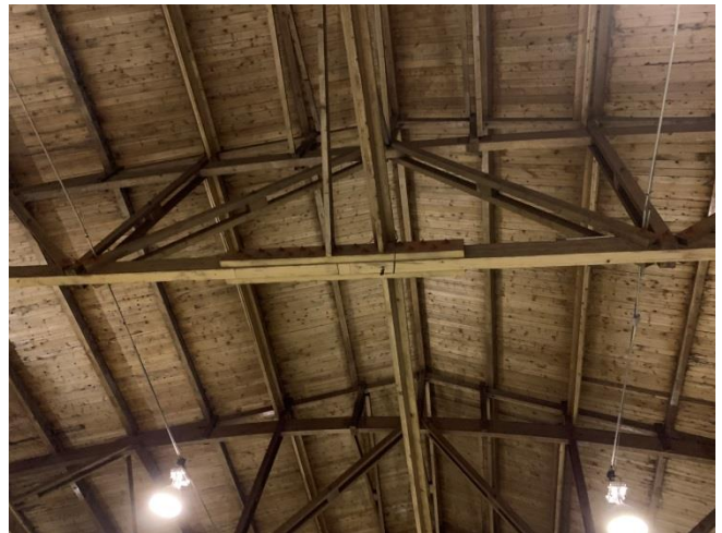
The roof support trusses were in fair to good condition.
