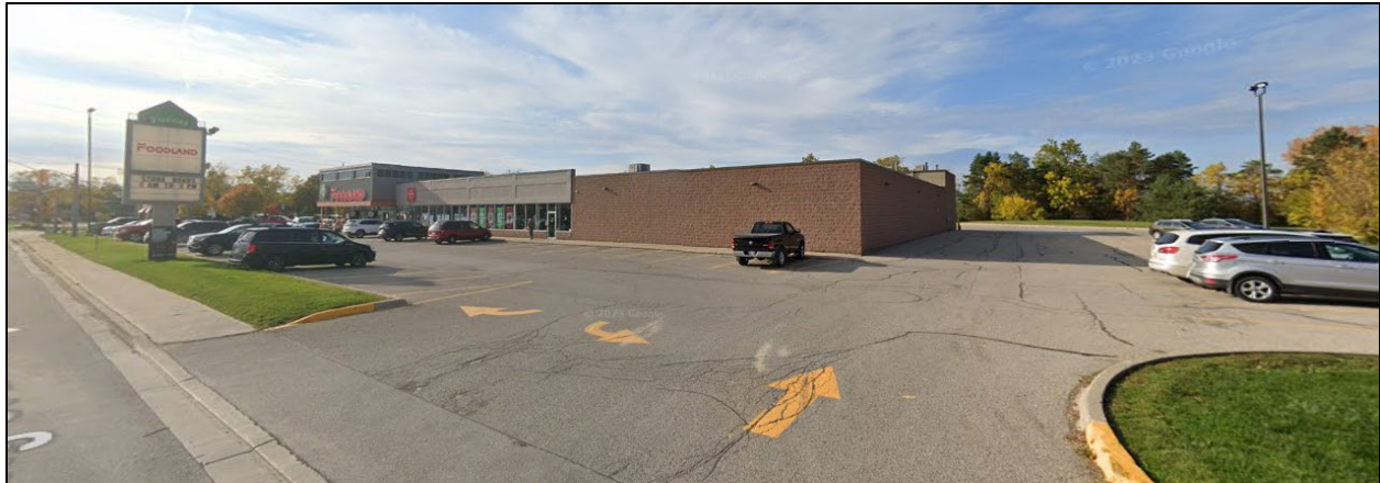
Image 2 – Subject lands, from King Street East
